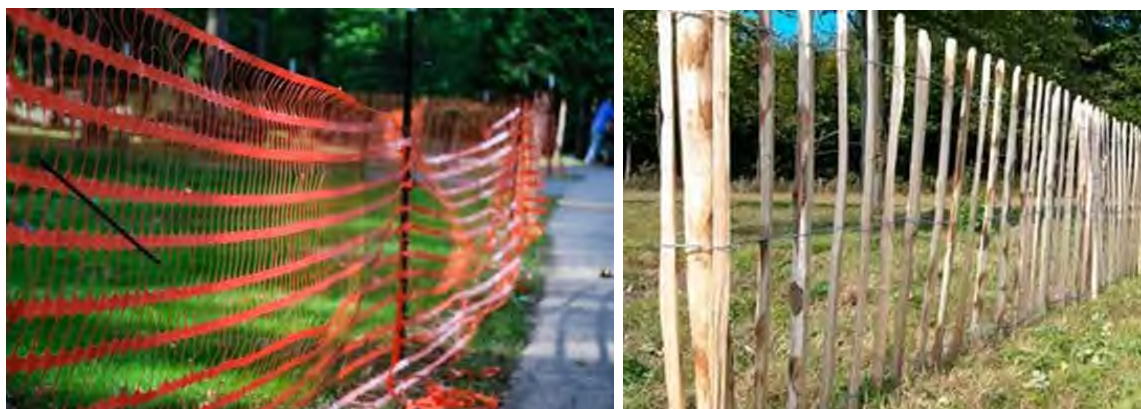
Figure C3 Tree protection fencing specification (Orange Weldmesh or Chestnut Pail)
